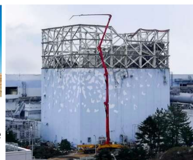
Pumping vehicles provided to Tokyo Electric Power for water injection after the Fukushima nuclear power plant accident
